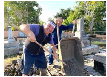
Stephen and Warren pouring cement in the cemetery.
