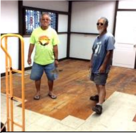
Chester & Larry removing the old floor tiles
